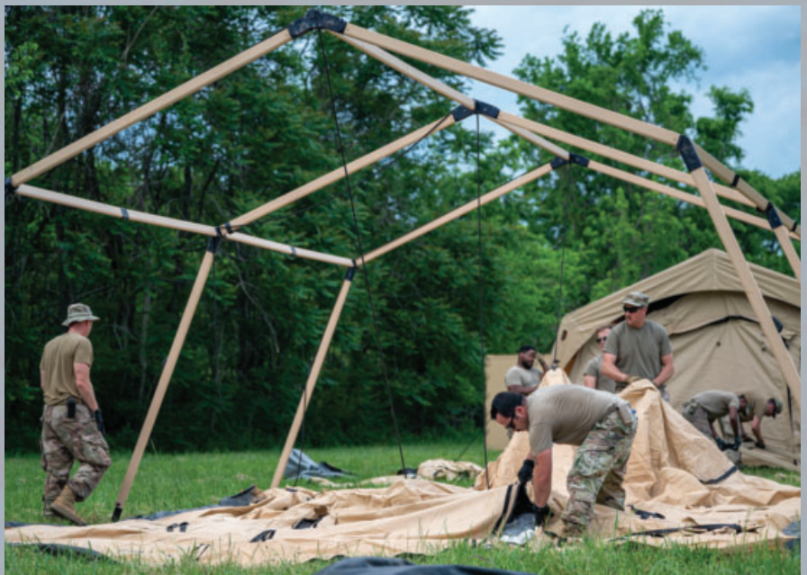
Members with the 27th Special Operations Wing Mission Sustainment Team Detachment 1 construct a tent during exercise Emerald Warrior 22.1 in Smyrna, Tennessee, May 5, 2022. The MST establishes forward-operating bases by providing initial site security, receiving cargo and personnel, and setting up shelter. Photo by U.S. Air Force Airman 1st Class Rachel L. VanZale.
